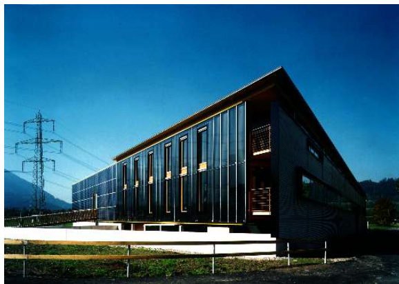
Thermal waste burning- / Photovoltaic- power station
